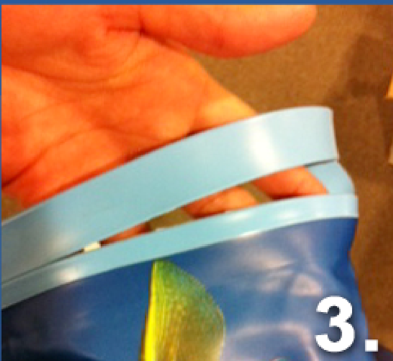
Bead After J-Hook is Removed
