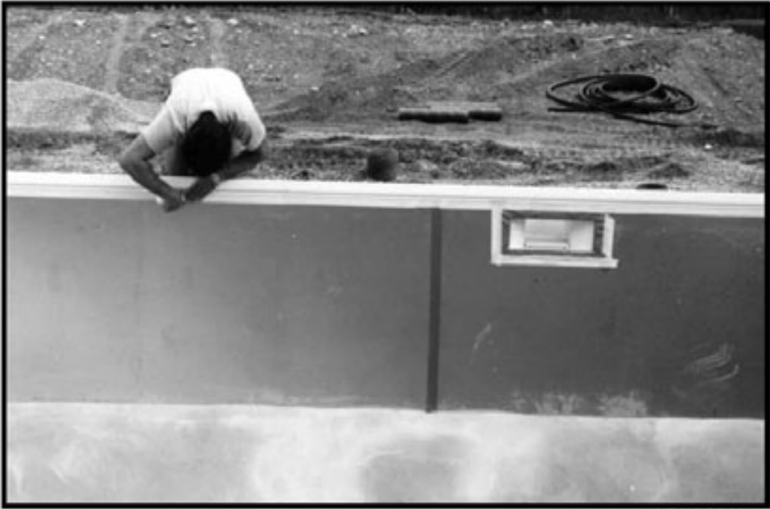
Tape off vertical wall seams.
