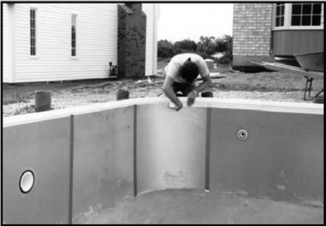
Tape around the perimeter of the coping.
